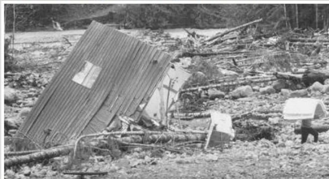
Alluvial fan debris flood damage on Canyon Creek, November 1990 (photo Bellingham Herald)
